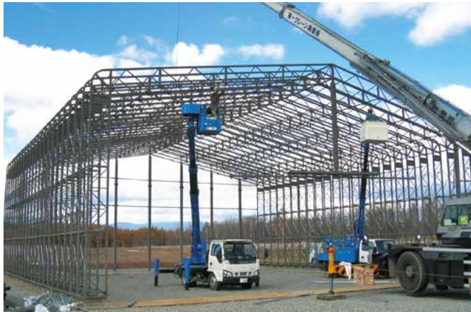
W:19.5 x L:20.13 (m) 積雪1m [敷鉄板] 施工状況
